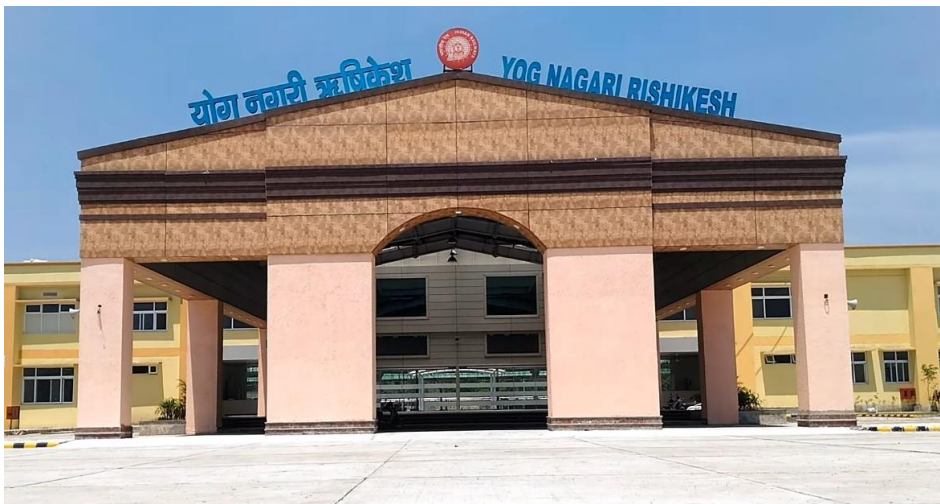
Figure 6:11 New Yog- Nagri Railway Station Rishikesh
