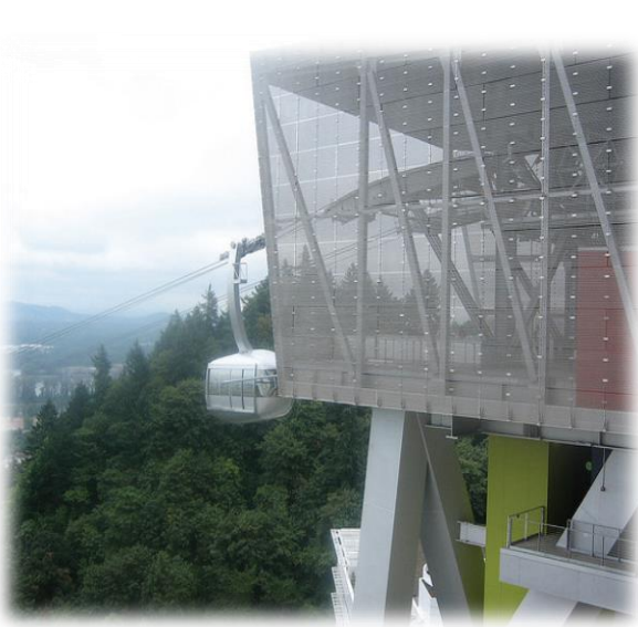
Vehicle arriving at Marquam Hill Station.
