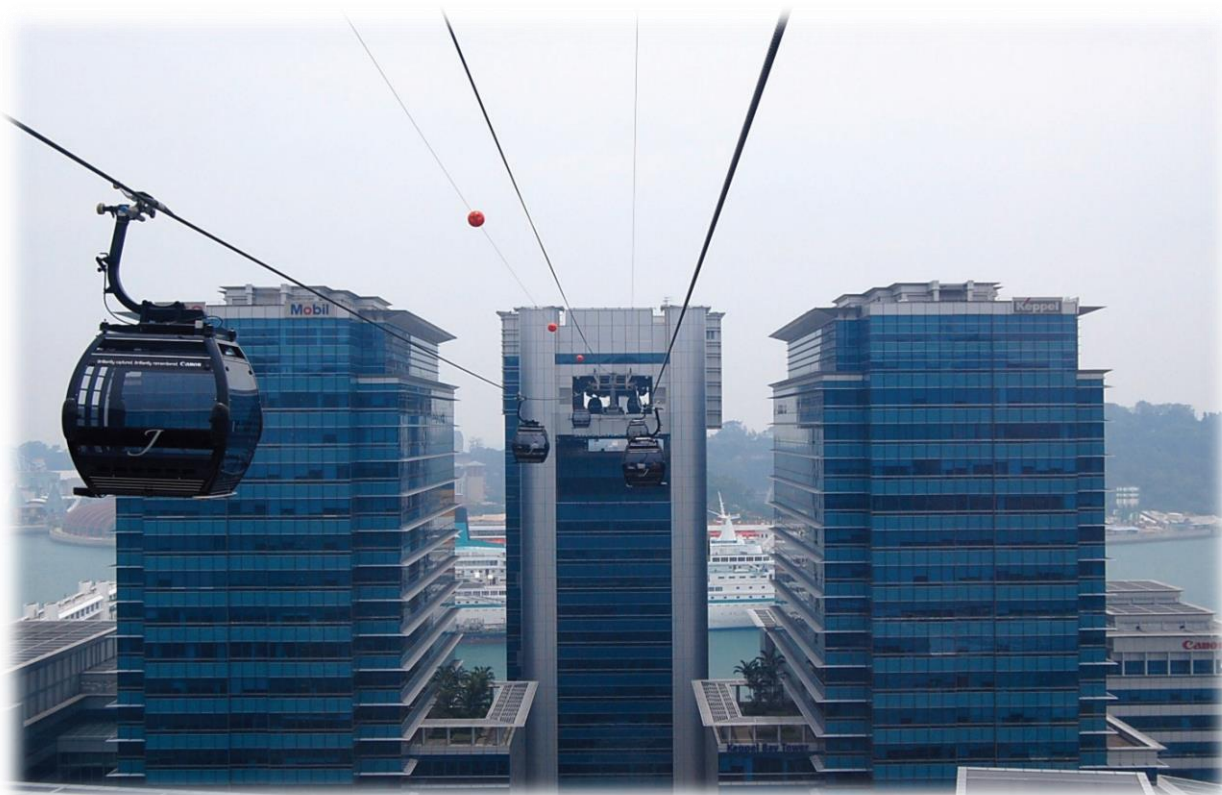
Entering the mid-station at Keppel Harbour Station, located inside an office building.
