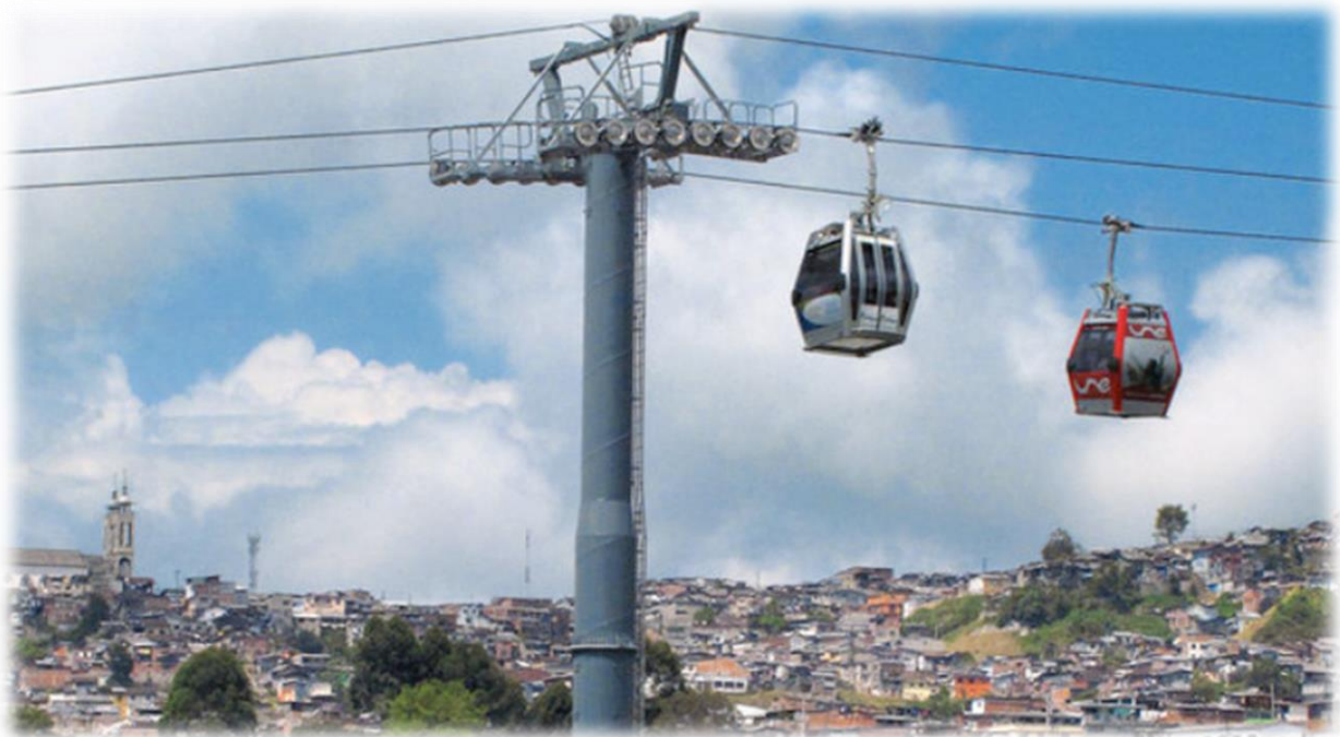
Tower Supporting a Ropeway System & Rope
